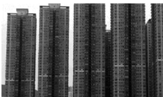
Figure 6: Tall buildings too closely pack together creating an 'effective' wind block to the city behind.
